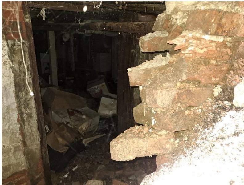
175 th E. 154 th Street (North Vaulted Sidewalk Area)
